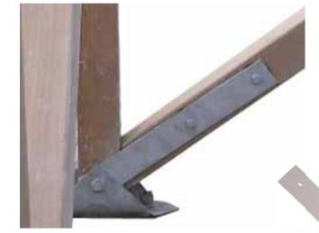
Cooling Tower Depot, Inc. offers a wide variety of Stainless Steel joint connectors. Our straps are available in both 304 and 316 grade stainless steel and offered in both three and five hole configurations.
